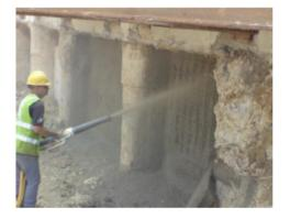
TamShot 10SS is used in sprayed concrete and annulus grouting applications which enables fast setting and/or where high early strength are required.
